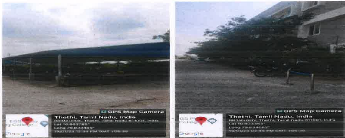
Figure 3. Roofed and Shaded Parking for two and four wheelers
