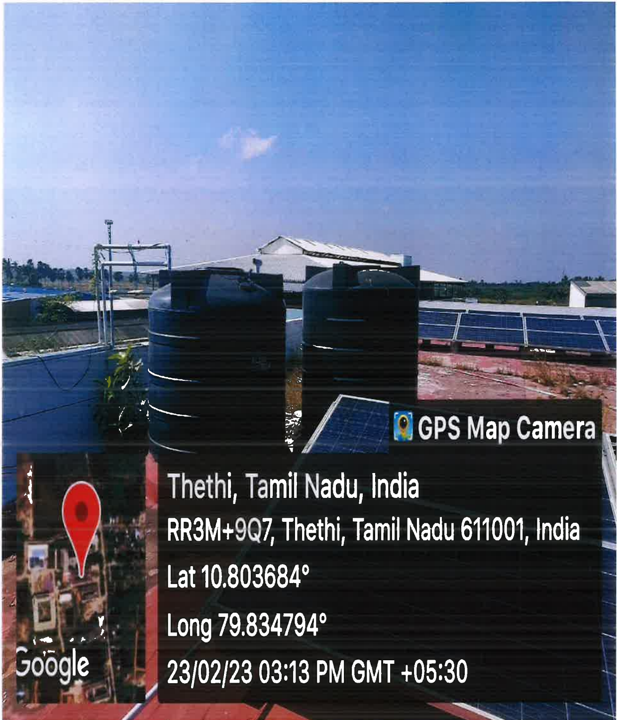
Construction of tanks and bunds (GG Block)
