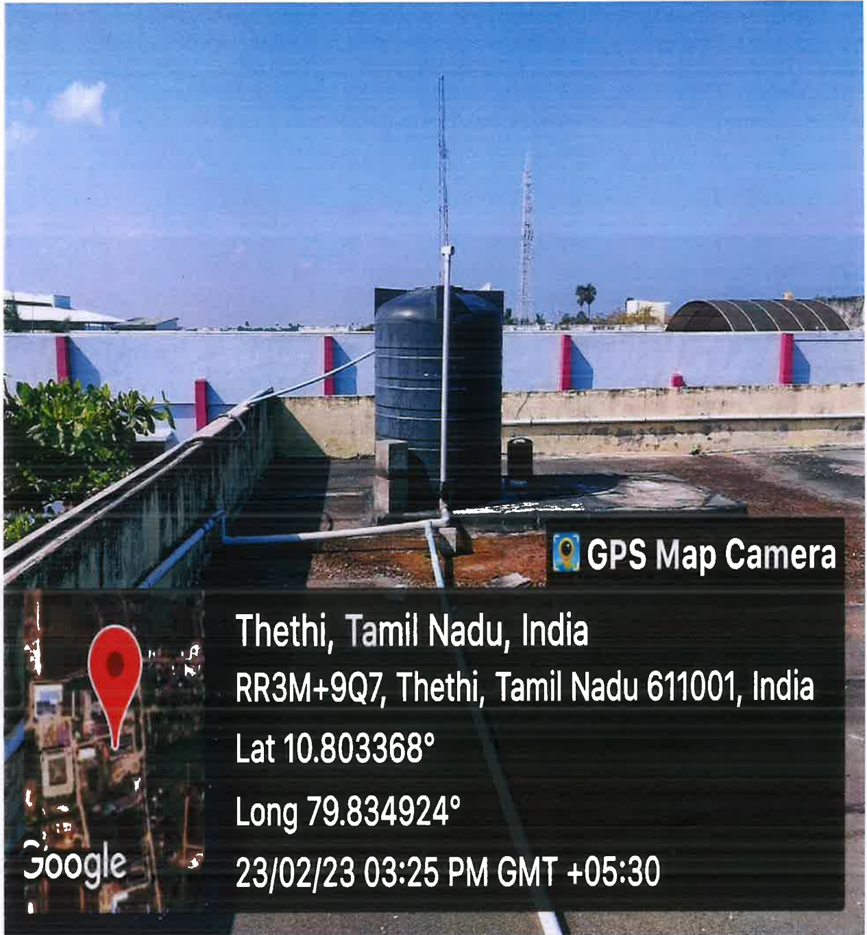
Construction of tanks and bunds (PG Block)
