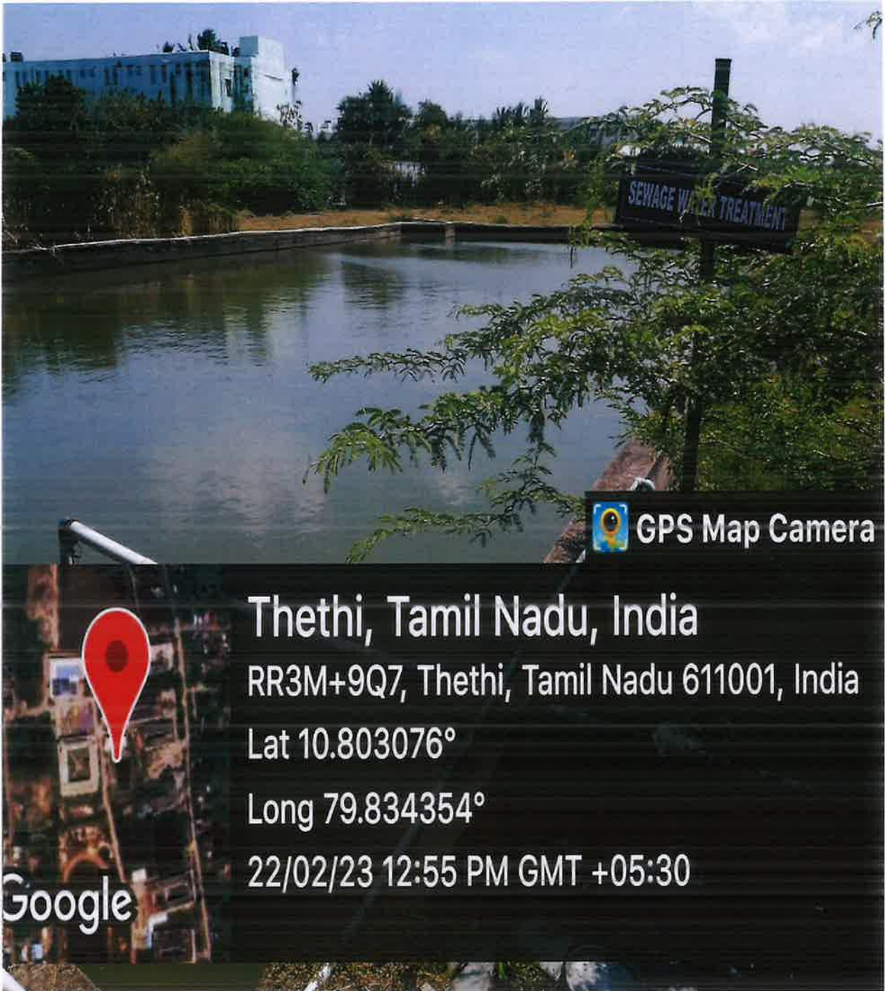
Sewage water treatment
