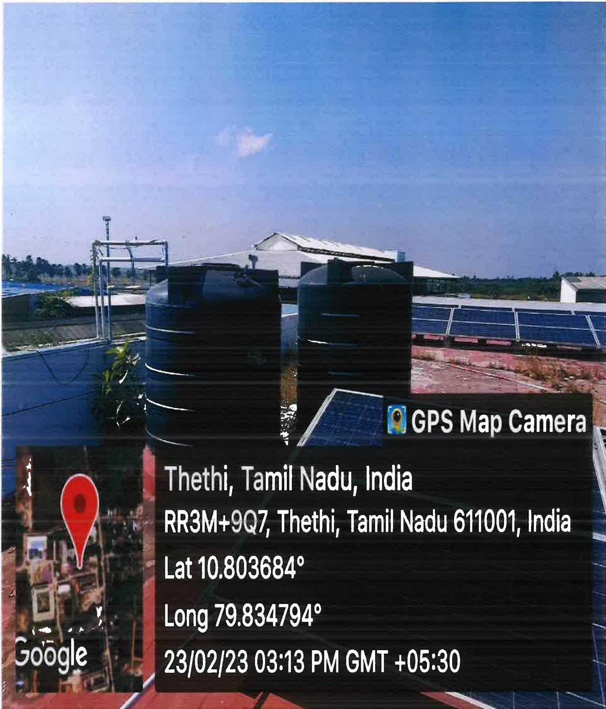
Construction of tanks and bunds (GG Block)
