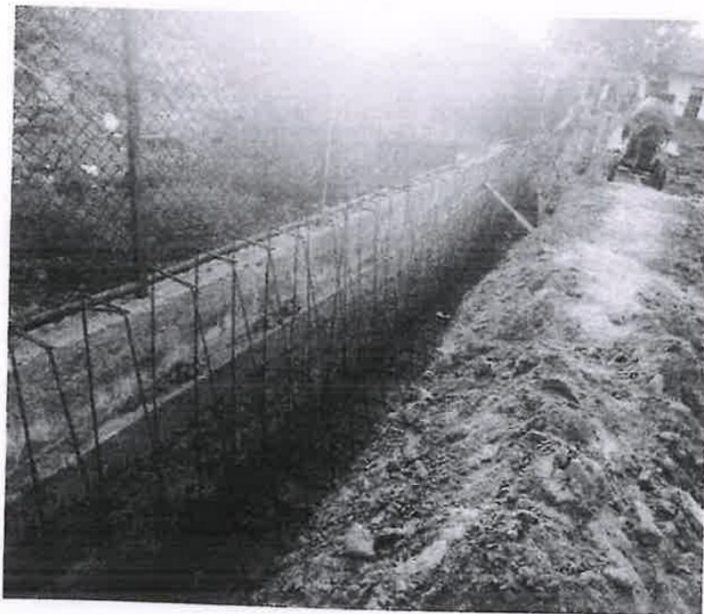
AFTER PCC REINFORCEMENT WORK
