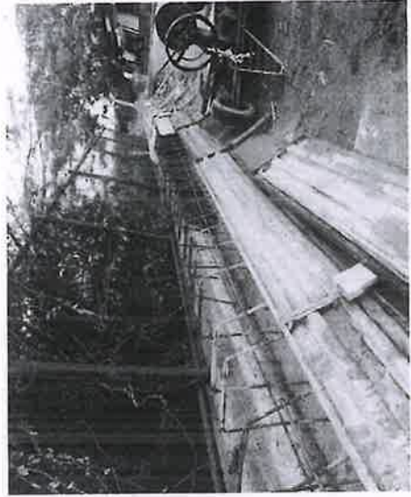
RETAINING WALL SHUTTERING WORK
