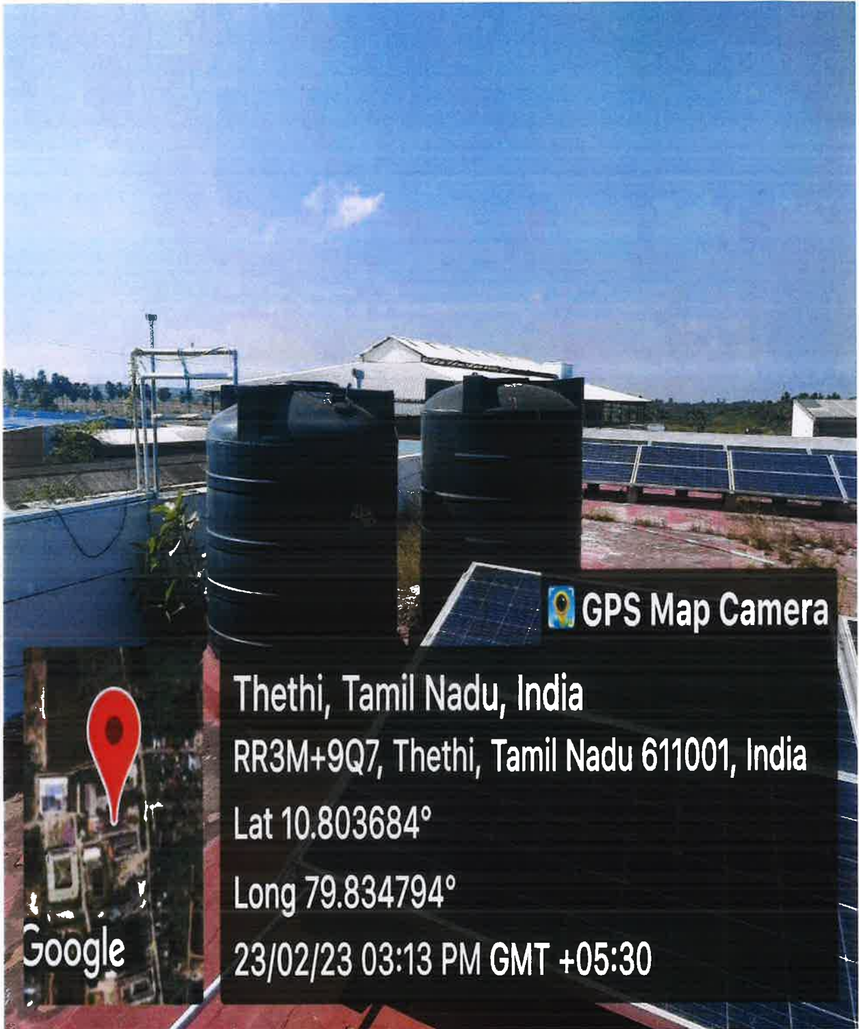
Construction of tanks and bunds (GG Block)
