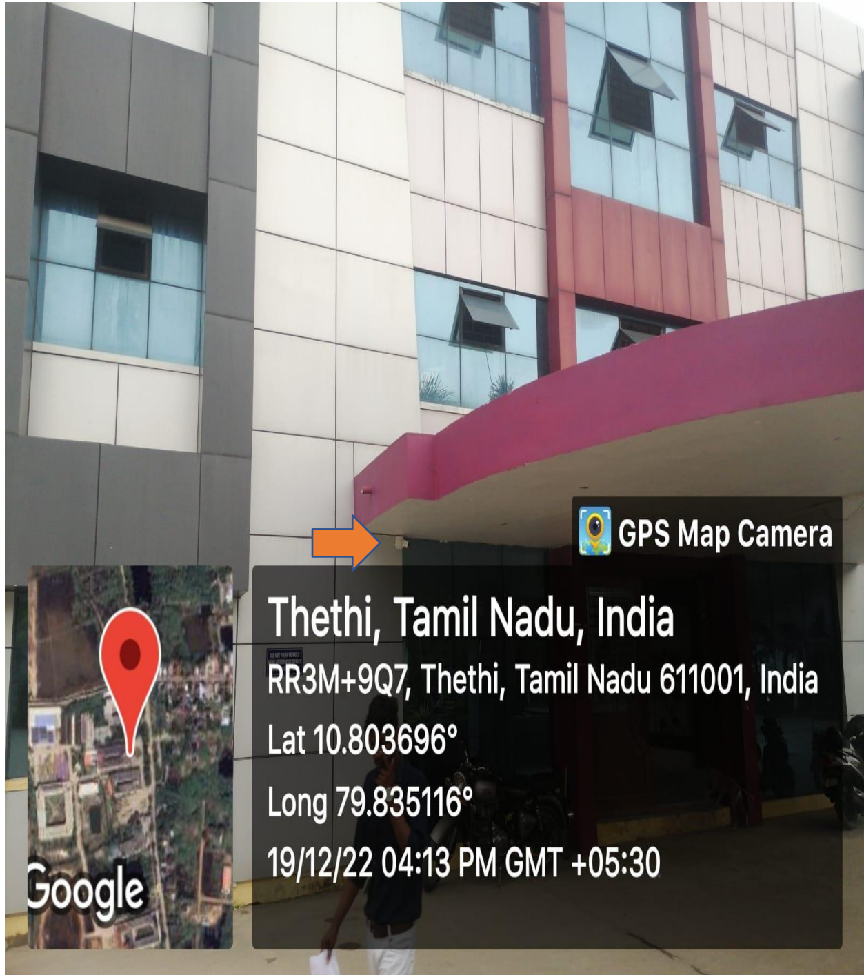
Outdoor CCTV Camera (GG Block)
