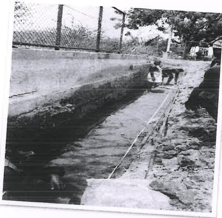
RETAINING WALL EARTH WORK
