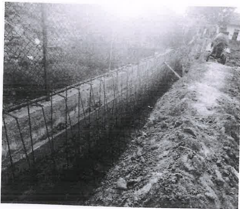
AFTER PCC REINFORCEMENT WORK
